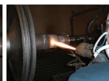
Turbine Shaft Repair
